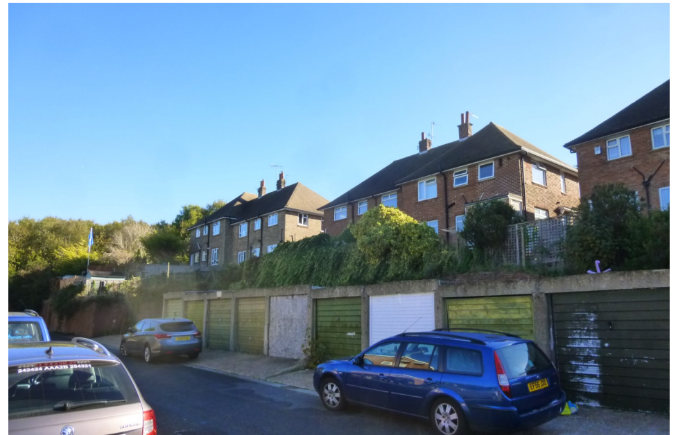
6. View of existing garages and rear of houses in Chichester Close
